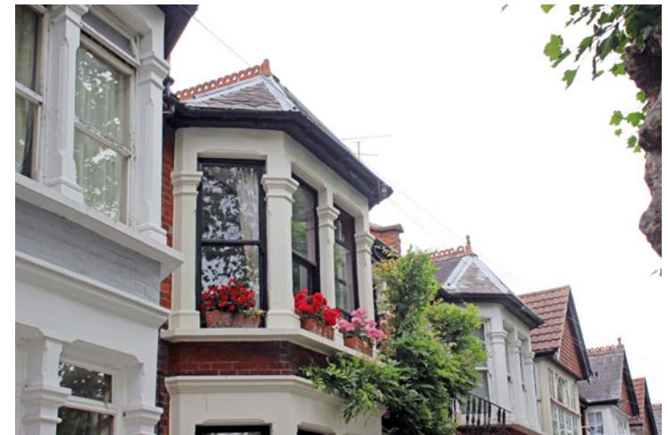
Hipped and gables roofs creating a lively skyline
