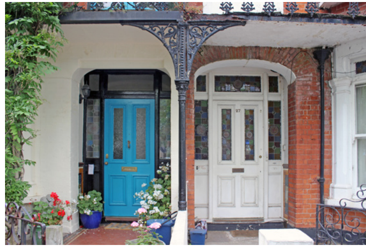
Recessed pair of porches with segmental arched entrances and original iron balcony and supporting structure (Nos.25 and 27)
