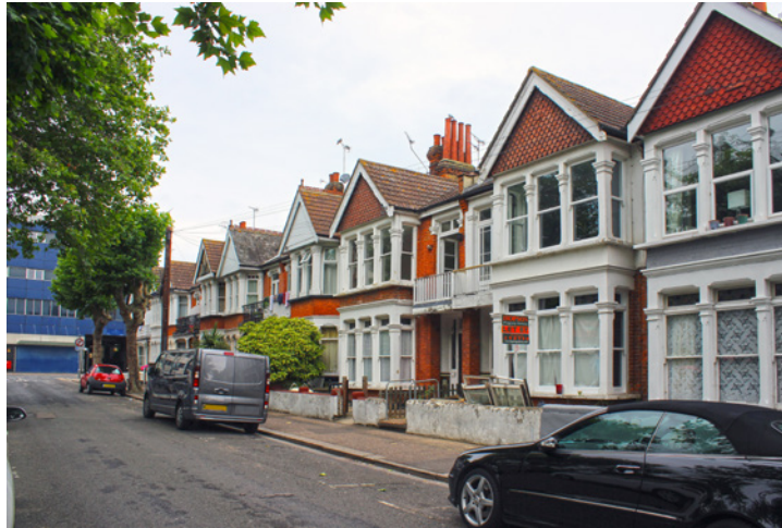
Later houses in the terrace, displaying Edwardian detailing
